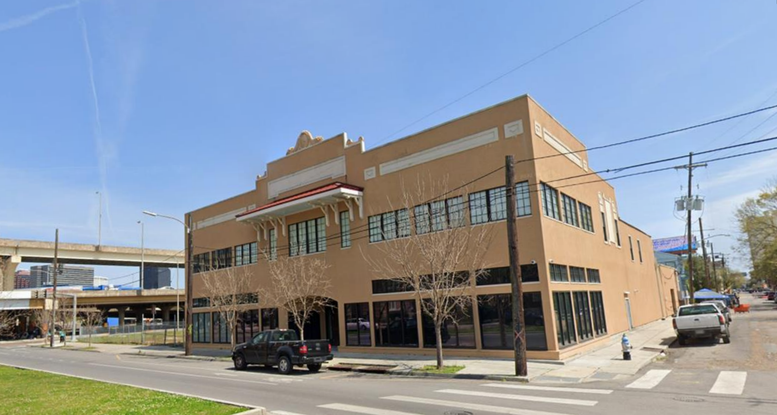
The New Orleans Mission Adaptive Reuse | Commercial | 28,000 sf
