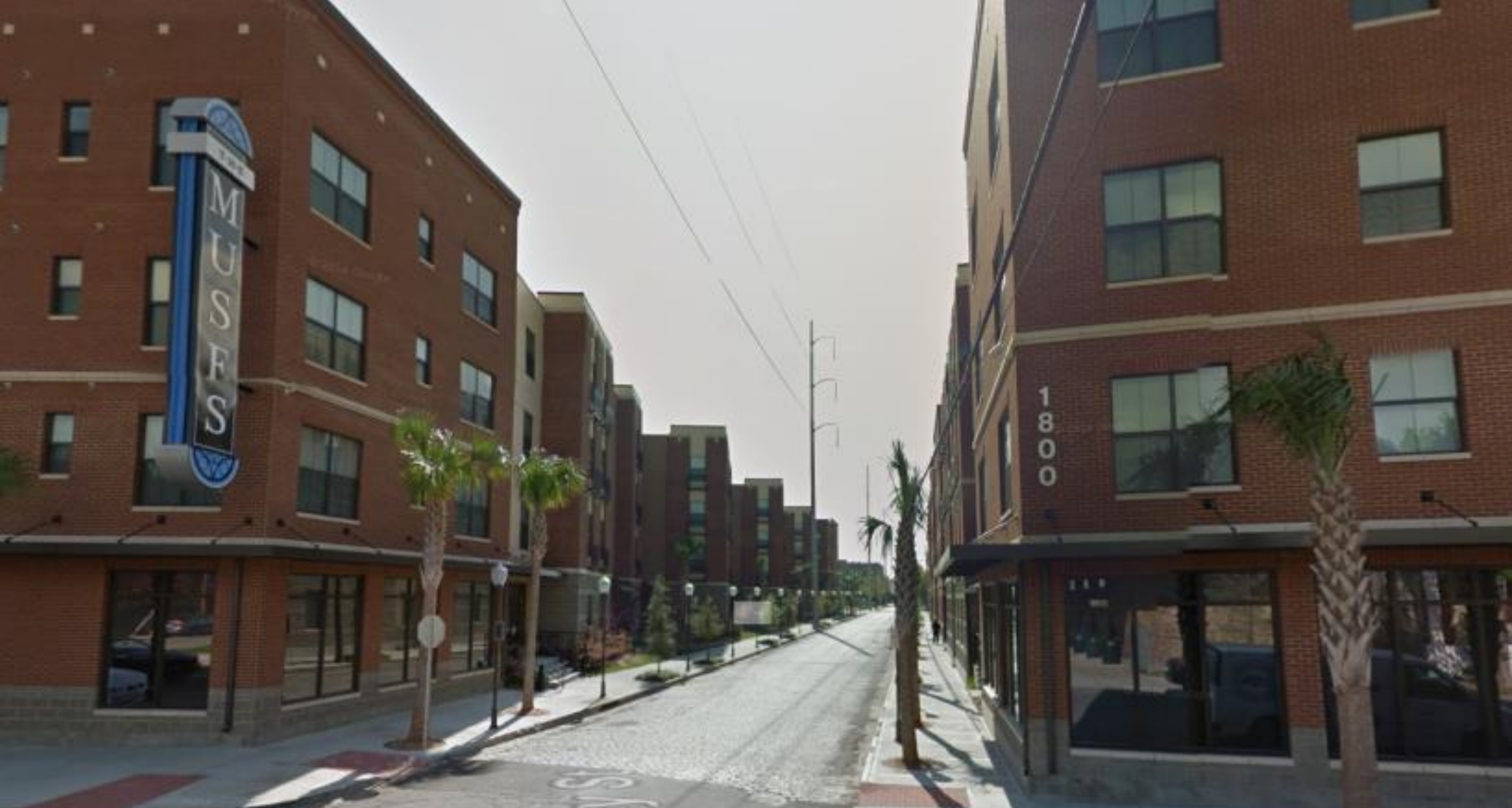
Muses I & II New Construction | Multifamily | 263 Units
